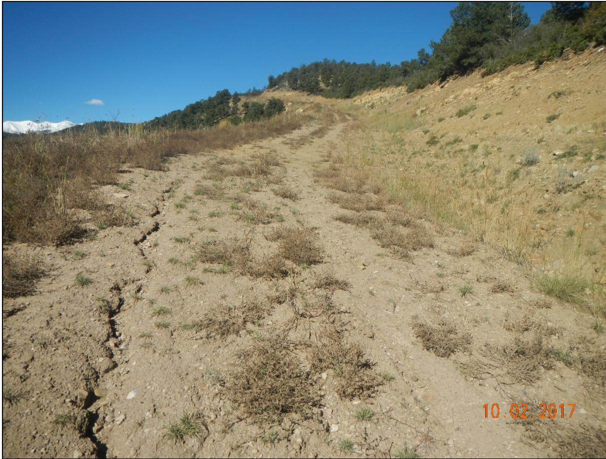
Photo 15. Facing northwest where the access road ascends the hillside. There are signs of erosion rilling occurring down the road.
