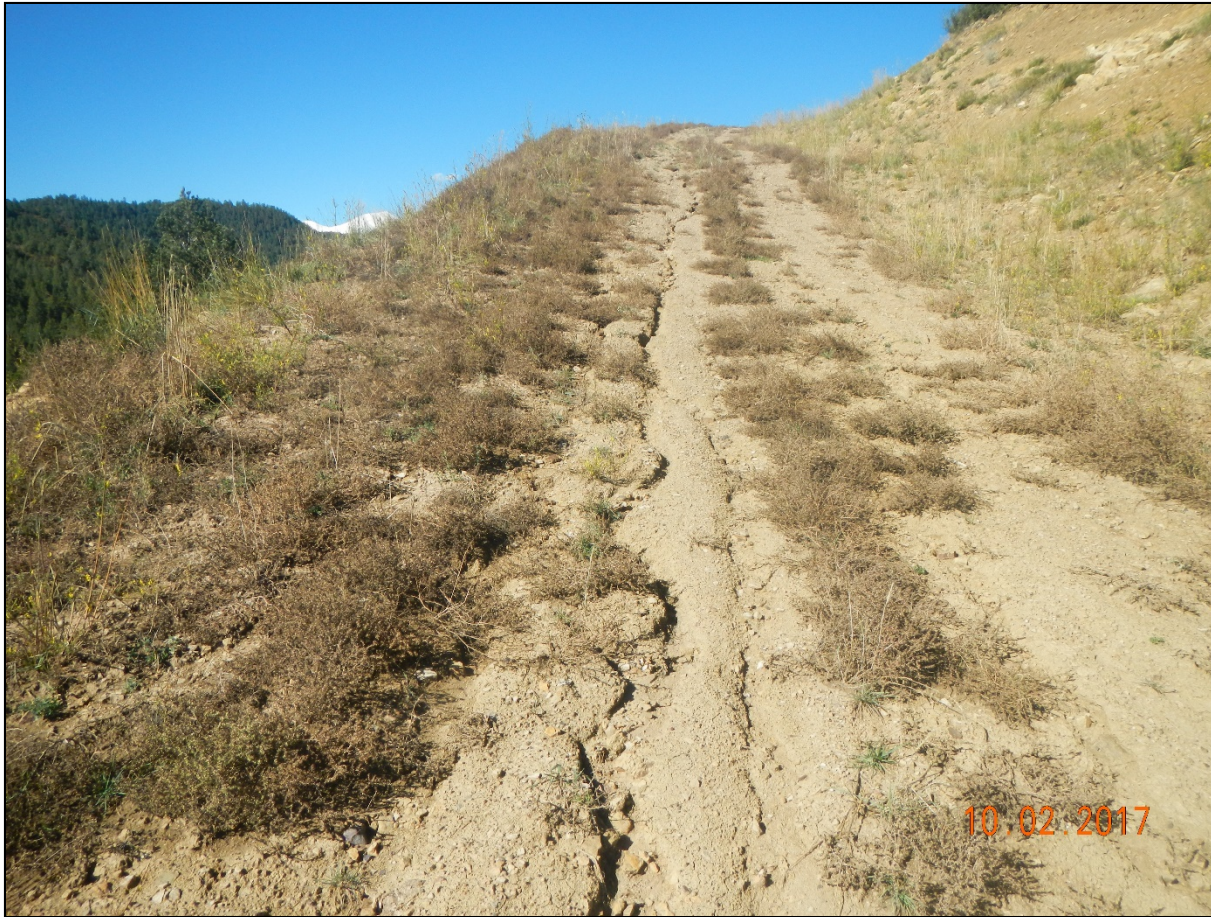
Photo 14. Facing northwest where the access road ascends the hillside. There are signs of erosion rilling occurring down the road.
