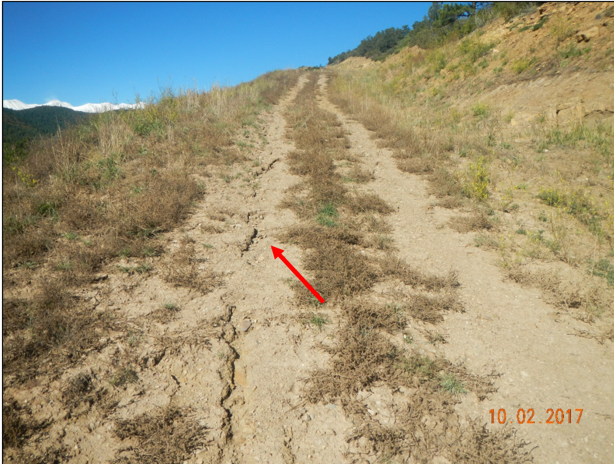
Photo 13. Facing northwest where the access road ascends the hillside. There are signs of erosion rilling occurring down the road.
