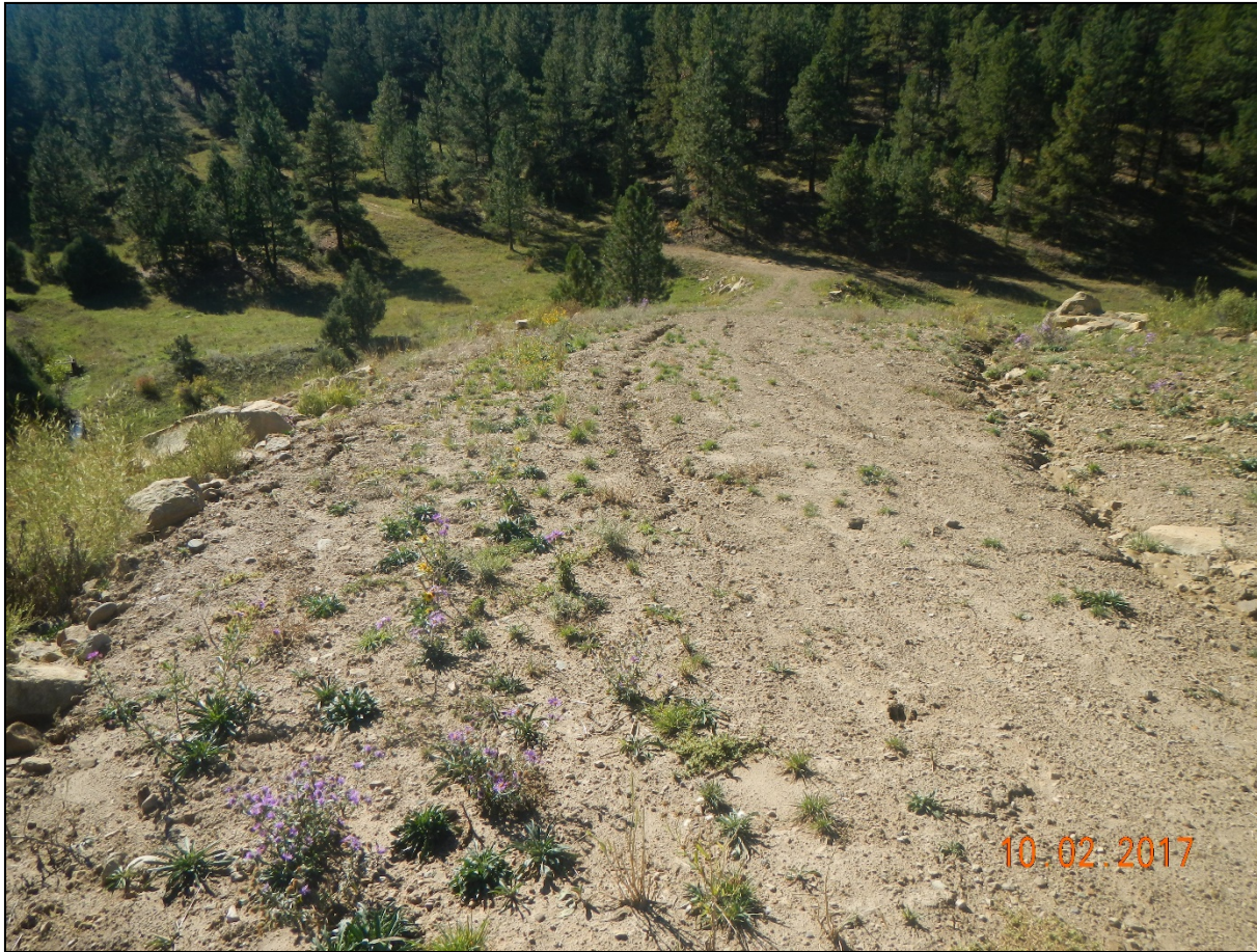
Photo 10. Facing south where the access road continues to the bottom of the canyon. There are erosion issues occurring down the road.
