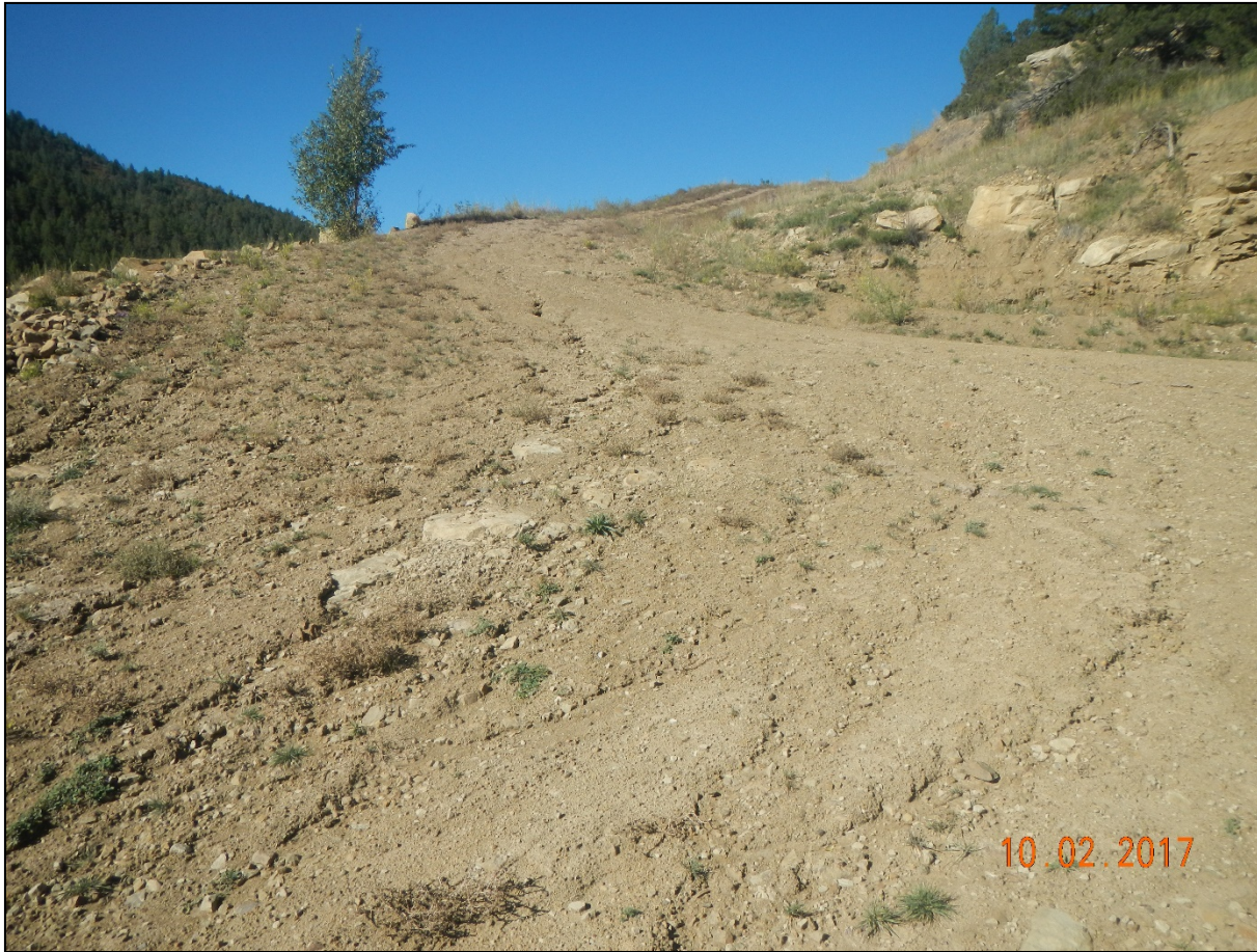
Photo 11. Facing northwest where the access road turns and ascends the hillside. There are signs of erosion occurring down the road.
