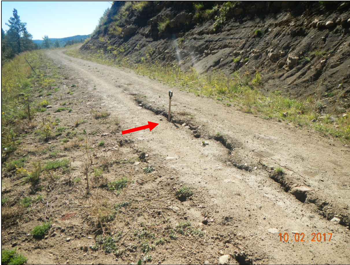
Photo 8. Facing southeast along the access road. There is signs of potential sloughing along the road. Arrow points to 3.5 ft. shovel placed into the surface opening.
