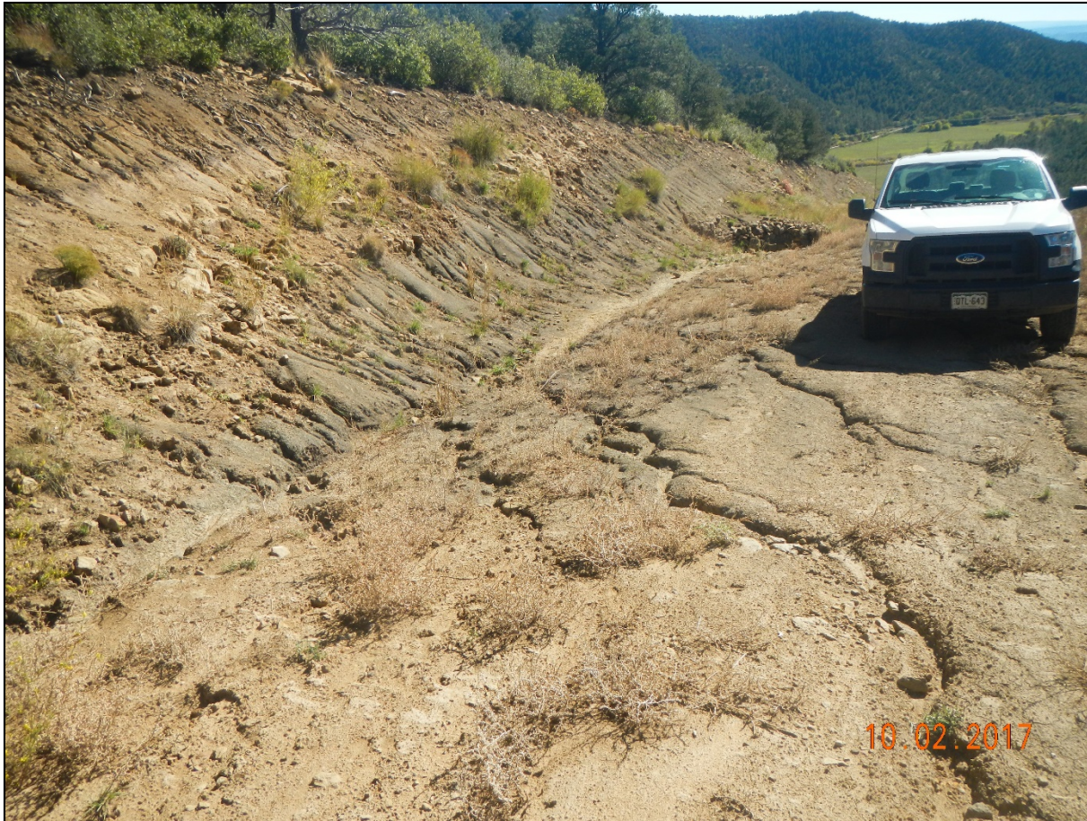
Photo 16. Facing back down the road. The cut slope is not adequately stabilized and there is erosion occurring down the road.
