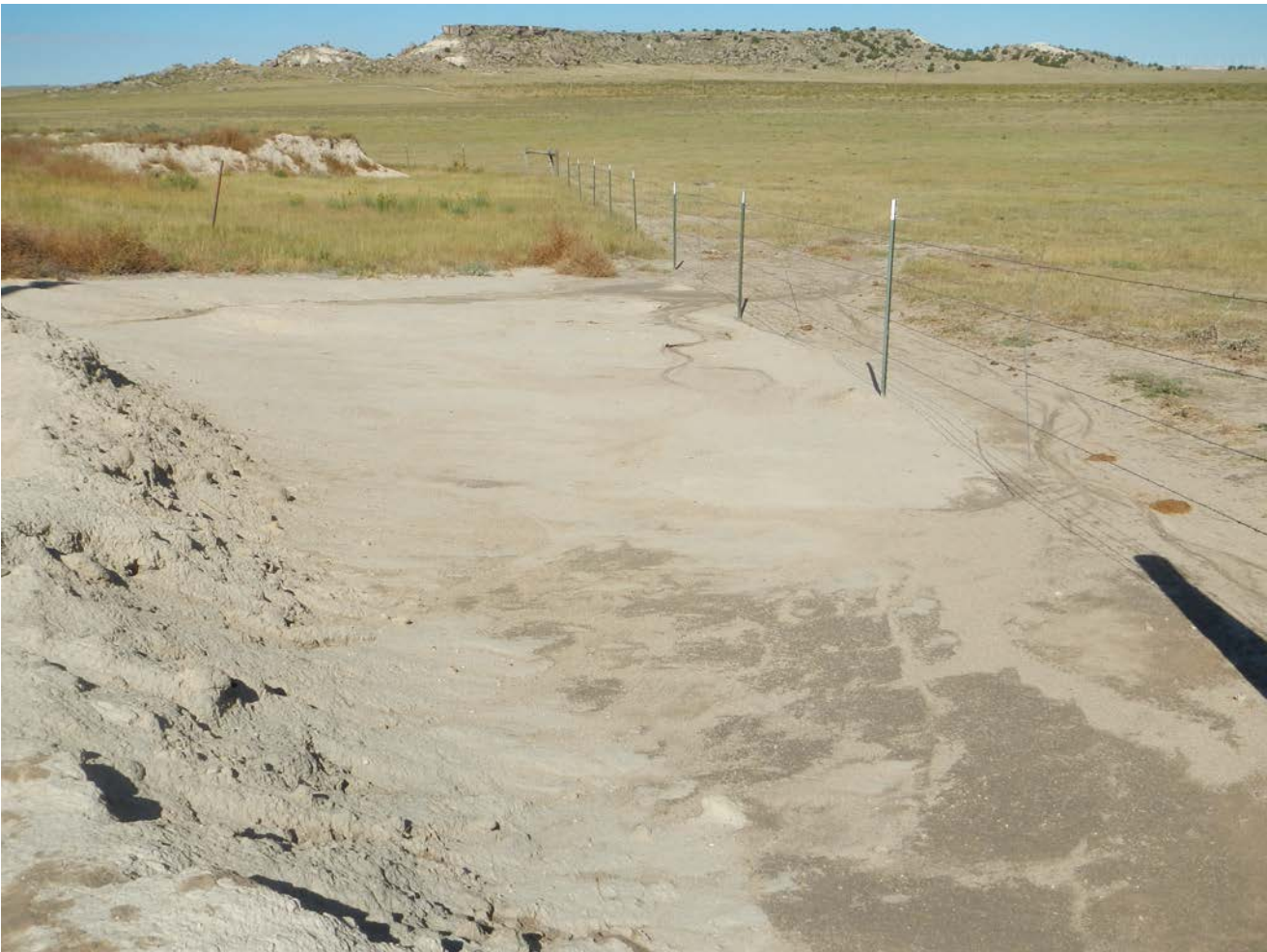
Area east of separator that needs erosion control BMPs to prevent off site sedimentation.
