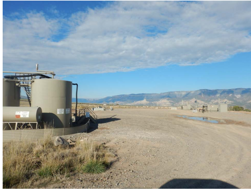
Location looking west
