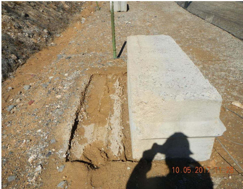
Deadman anchor dragged towards pit. Looking NNW
