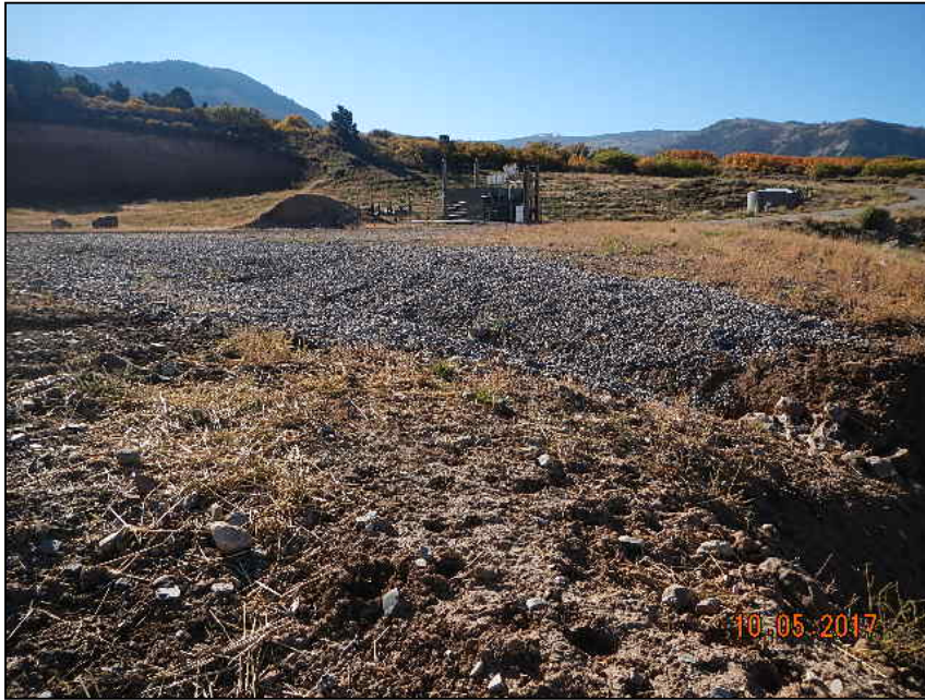
Photo 1. Gravel has been added to area of erosion on pad surface and sediment trap maintained.
