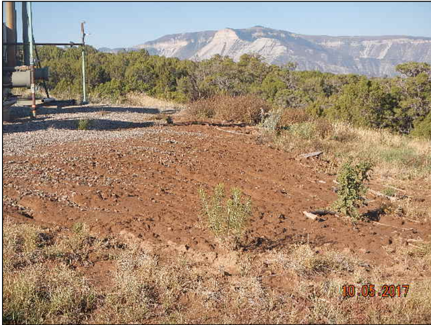
Photo 1. Rilling and erosion behind separators.
