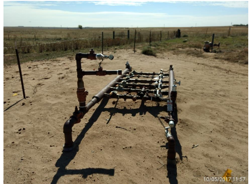
Flow line manifold. Unidentified riser 39.917841, - 104.732105
