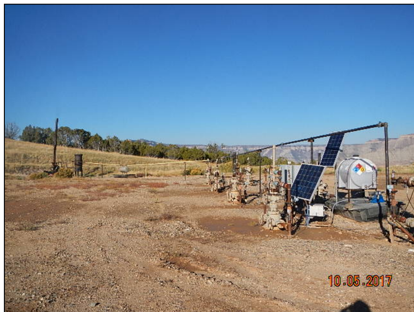
Photo 1. Field flare and ECU onnected to the 11-11, 11-12, and 11-12BB wells.
