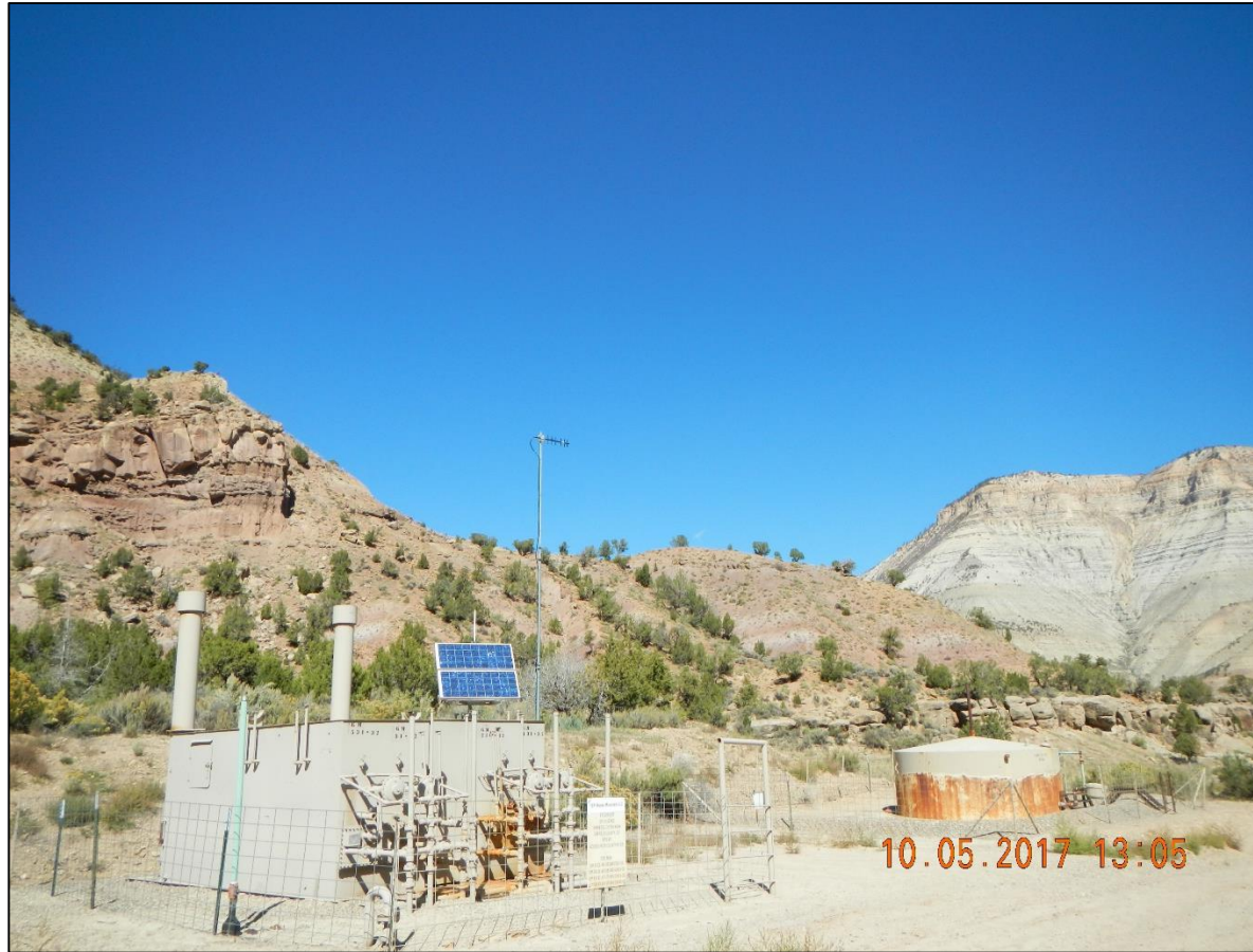
Tank battery and separators
