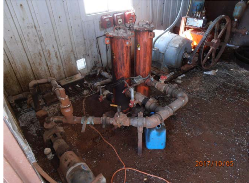
Photo 12: Leaks inside injection pumphouse.
