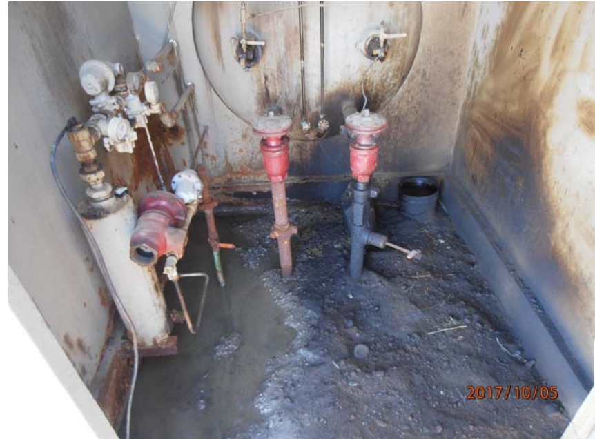
Photo 6: Oily soil inside horizontal treater shed.
