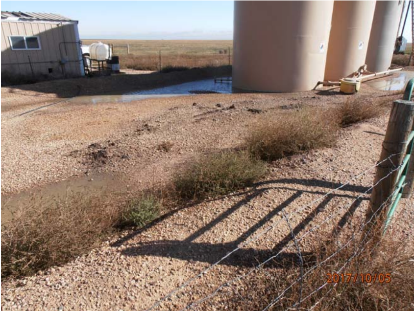
Photo 1: Oily soil in tank battery. Standing water is stormwater.
