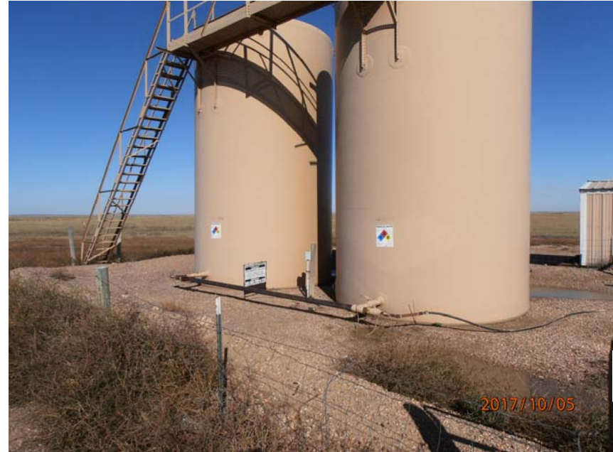
Photo 2: Produced water ASTs.
