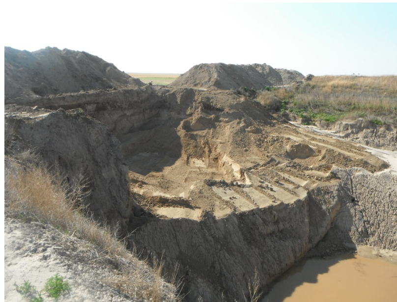
Skim pit and evaporation pit after removal of shared wall
