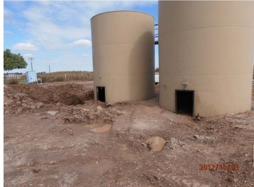
Photo 4: Tank Battery decommissioning in progress.
