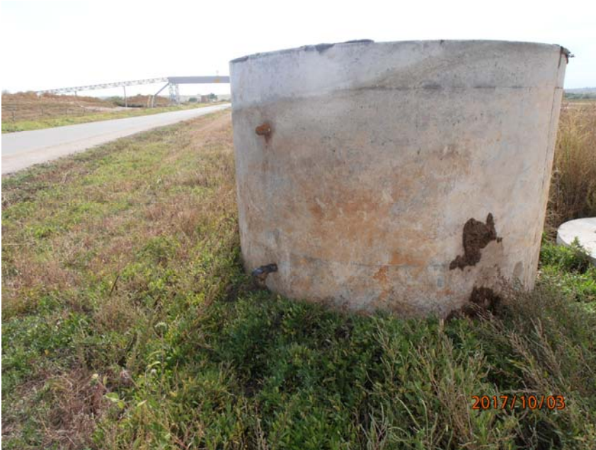
Photo 3: Partially buried produced water vessel removed from excavation and staged onsite.
