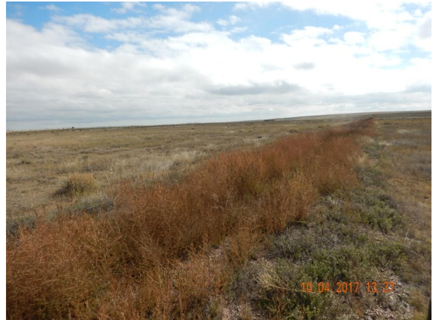
Photo 2. Photo taken from a portion of the access road, facing South. Russian thistle growing throughout the access road portions of the road, gravel still on access road, and access road has not been contoured or seeded.
