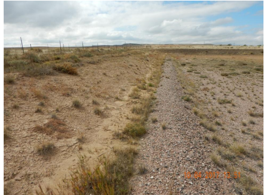
Photo 12. Photo taken from the southern location, facing West. Operator has not performed reclamation as cut slopes and gravel are evident throughout the location.
