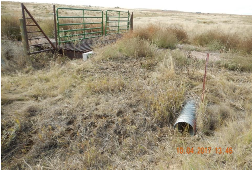
Photo 5. Photo taken from the entrance of the location, facing West. Culvert, cattle guards, and fence have all been left at location.
