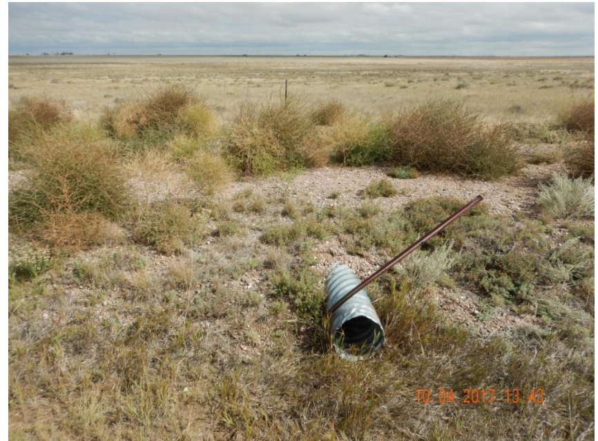
Photo 4. Photo taken from another portion of the access road, facing East. Culverts need to be removed per Rule 1004.
