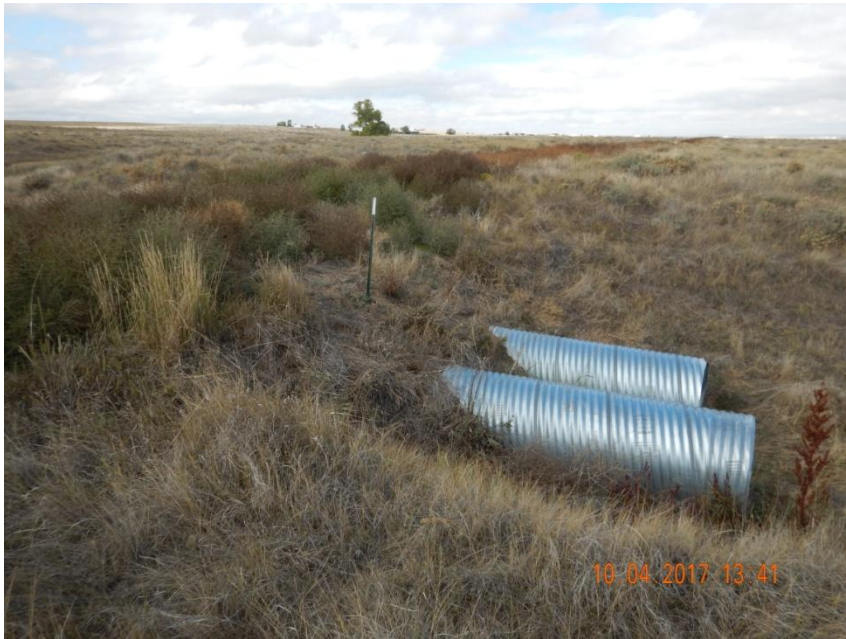
Photo 3. Photo taken from a portion of the access road at an intermittent stream crossing, facing North. Culverts need to be removed per Rule 1004.
