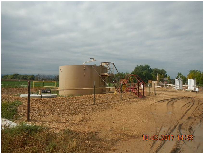
SHARED TANK BATTERY TAKEN FROM THE SOUTH THIEF HATCH AND BLOW DOWN VALVE CLOSED
