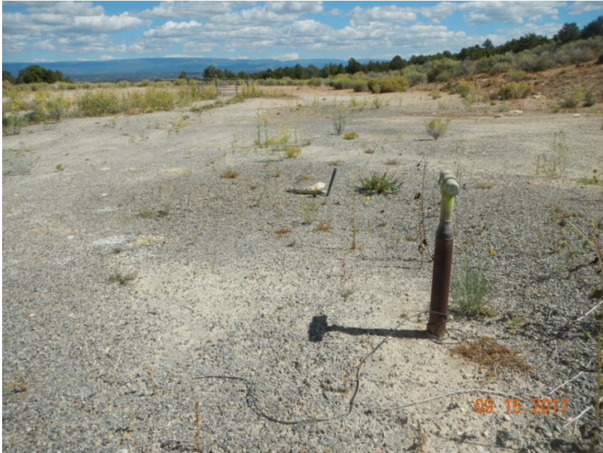
Photo 7: View of unmarked risers on the well pad.
