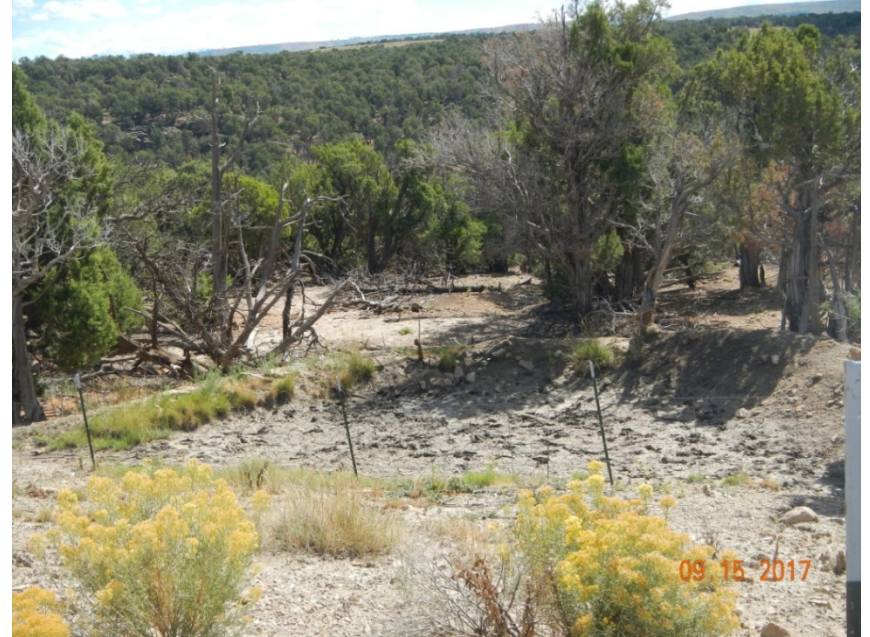
Photo 6: View of silt trap in the southwestern corner of the project area. This is almost full of sediment and will soon require maintenance.
