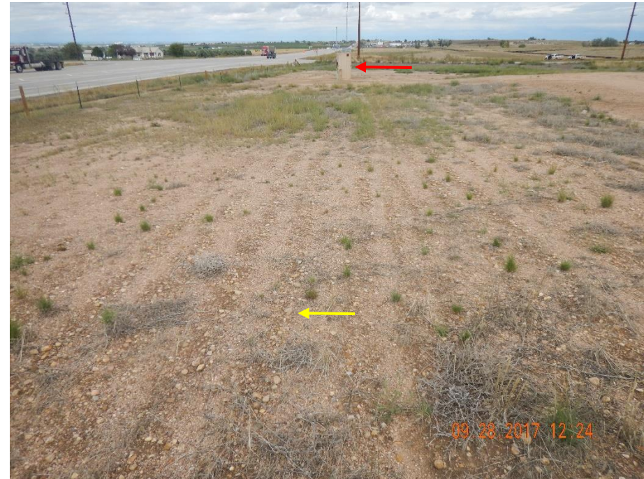
Photo 4: Photo taken from the south end of the former tank battery location, facing south. Red arrow indicates meter shed equipment remaining. Photo shows areas of the battery where striations in the soil are evident, indicating reclamation activities appear to have been attempted at one point prior to the inspectors previous visits. However, gravel remains and if any revegetation activities have been conducted, they have been unsuccessful.
