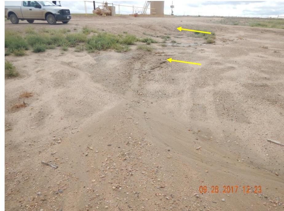
Photo 2: Photo taken from the former battery location, facing southeast towards the active Broomfield tank battery. Photo shows stormwater runoff from the active battery is causing erosion degradation on the slopes, as well as erosion degradation at the former Freedom tank battery. COGCC rule 1002.f requires stormwater management until final reclamation has passed.
