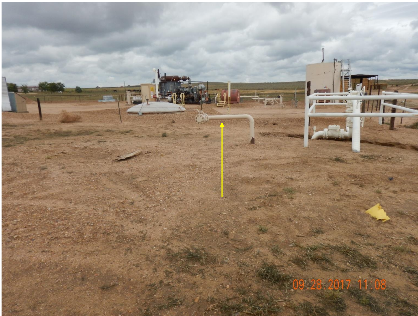
Photo 3: Photo taken from the former battery location, facing north. Inspection doc. #675103866 noted that the meter sheds had been removed, but pipe riser equipment associated with the meter sheds still remain. Photo shows riser equipment has not been removed per the corrective actions.
