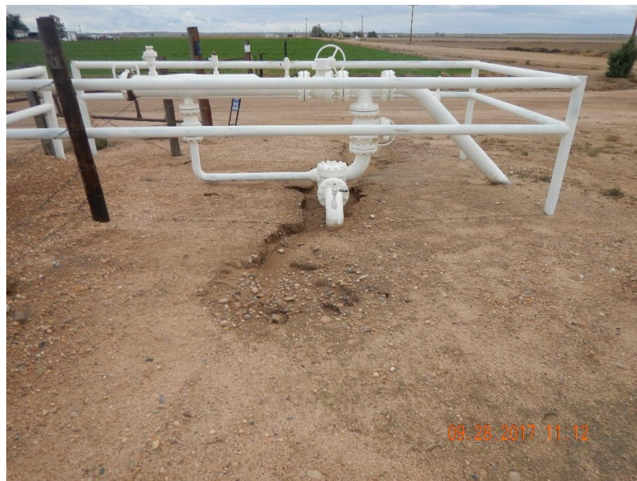
Photo 2: Photo taken from the northeast end of the battery location, facing east. Photo shows stormwater erosion degrading the location.
