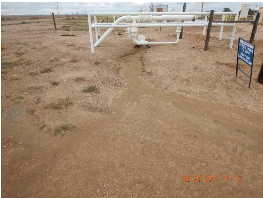
Photo 1: Photo taken from the northeast end of the battery location, facing west. Photo shows stormwater erosion degrading the location.
