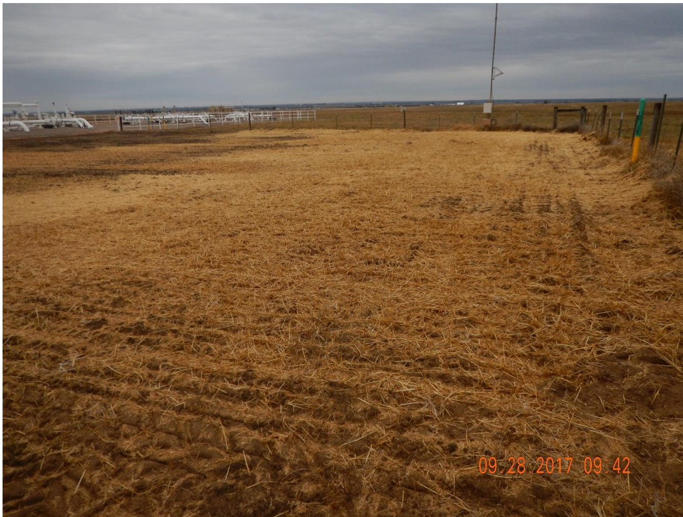
Photo 1: Photo taken from the southwest end of the former battery facility. Photo shows meter houses have been removed and area appears to have been re-seeded and crimped with straw for stabilization.
