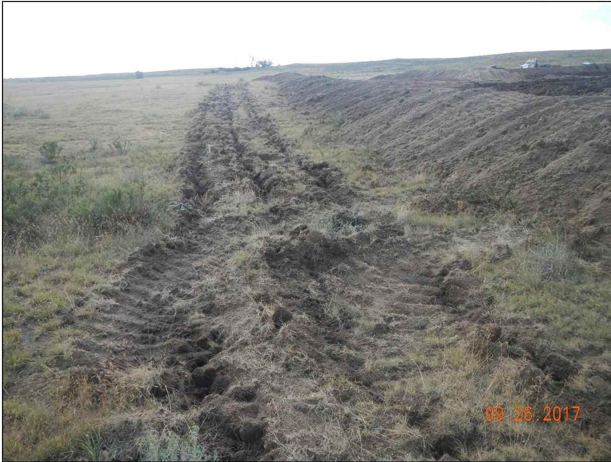
Photo 6. Facing south along the east side of the location. A soil berm is constructed around the perimeter and surface roughening has been created around the perimeter.
