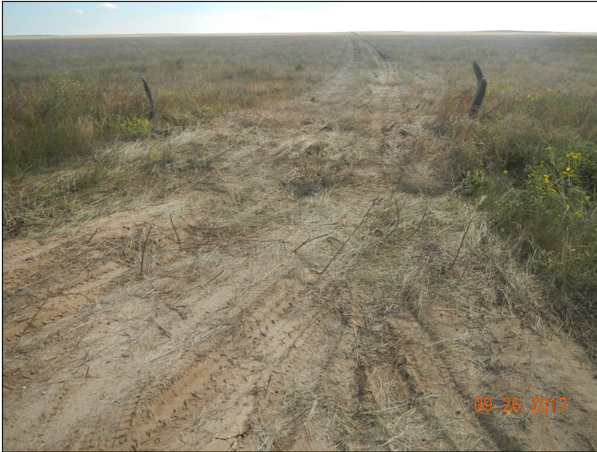
Photo 1. Facing east at the beginning of the access road. Contractor was preparing to install tracking pad. Operator must ensure tracking pad is installed to prevent sediment tracking onto county road.
