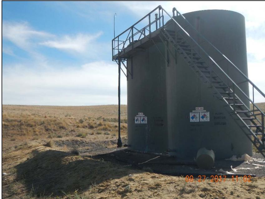
Photo 2. Tanks labeled with produced water and condensate as contents.
