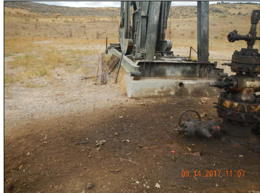
Photo 4. Close-up of stained soil at wellhead.
