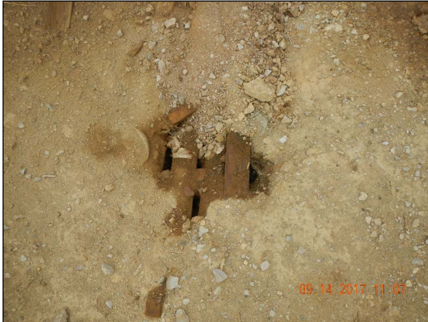
Photo 5. Partially covered rathole with fluid present.
