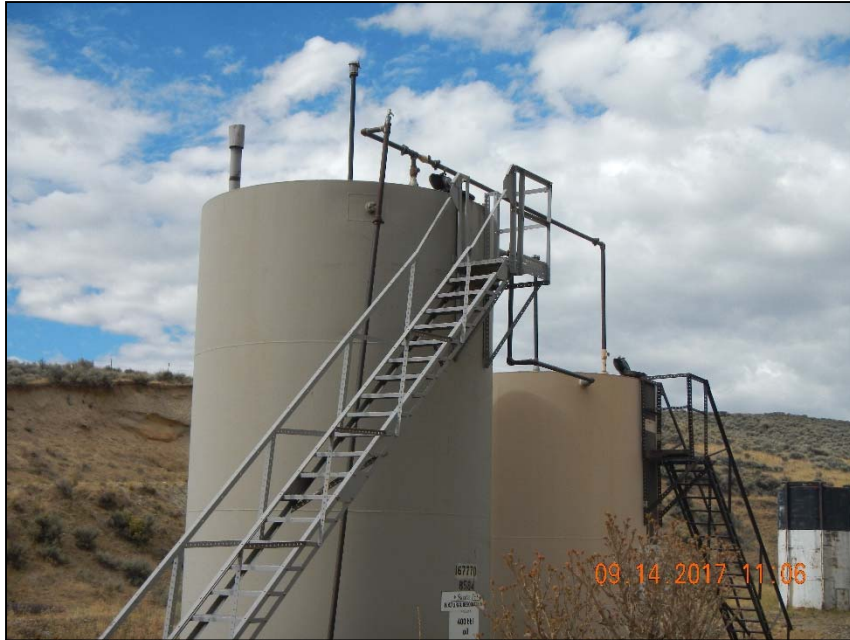
Photo 7. Gauge hatches open on both tanks.
