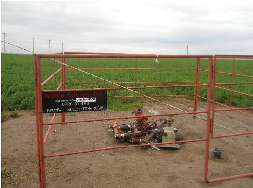
**Wellhead looking west. Well has been PA, waiting for SC to be cut/removed along with wellhead equipment.**
