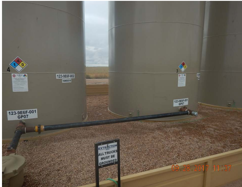
Photo 3: No capacities on production tanks
