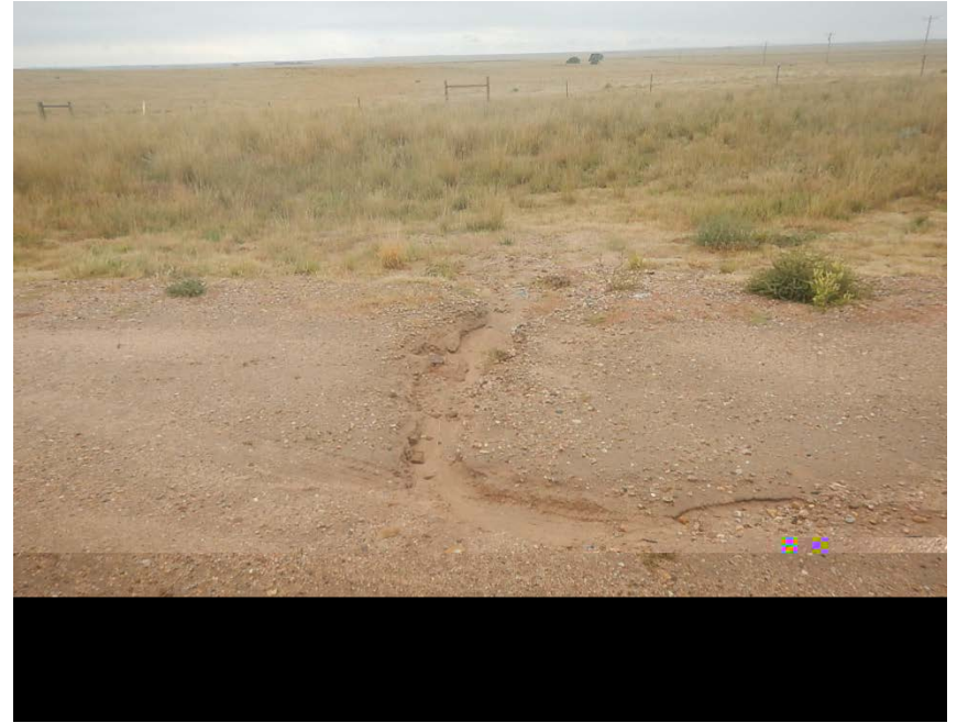
Photo 6: Stormwater erosion on S side of location
