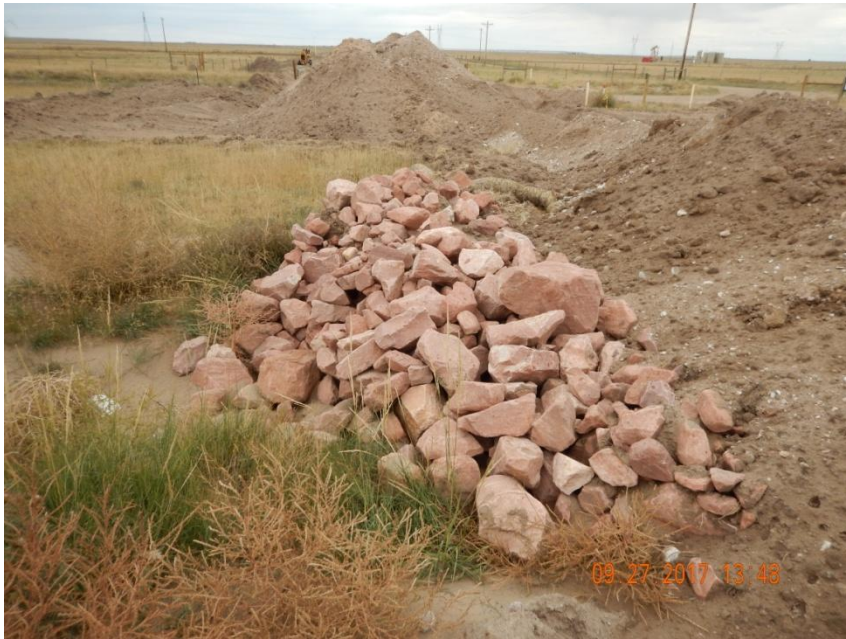
Photo 1. Photo taken from the southeast location, facing East. Appears Operator may have installed a sediment trap but pipeline disturbance has damaged BMPs.
