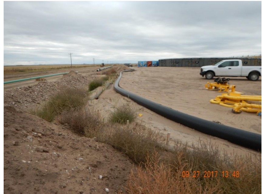
Photo 2. Photo taken from the southeast location, facing West. Photo illustrates pipeline construction and disturbance. Temporary BMPs (straw wattles) appear to be installed between the water line and the unconsolidated soil material.
