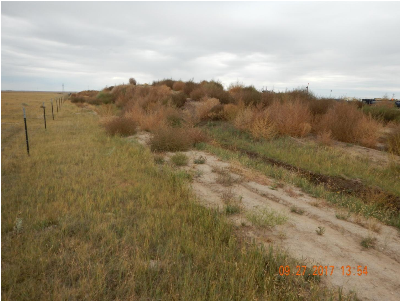
Photo 6. Photo taken from the western topsoil stockpile along the north-facing side, facing East. Russian thistle has established throughout the stockpile which is not protective of topsoil per Rule 1002.c. and Russian thistle is considered weed debris which needs to be controlled per Rule 603.f.
