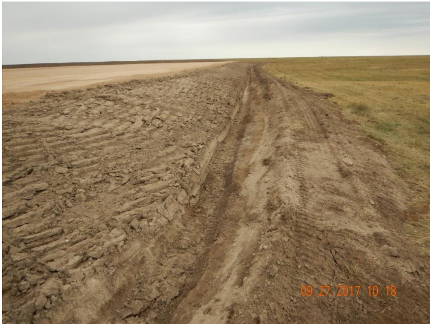
Photo 3. Photo taken from the southeast location, facing North. Temporary BMP's (ditch and berm) have been installed.
