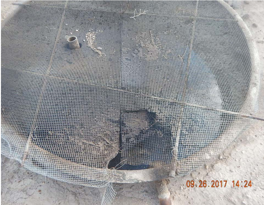
Photo 3: Gap in mesh on open top skim
