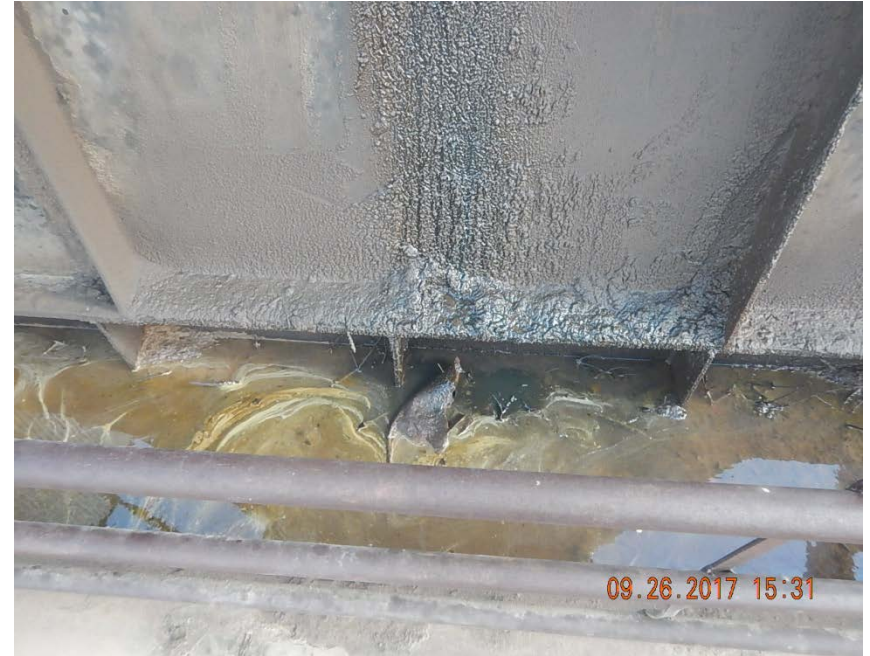
Photo 8: Stained soil, oily fluid at pump jack
