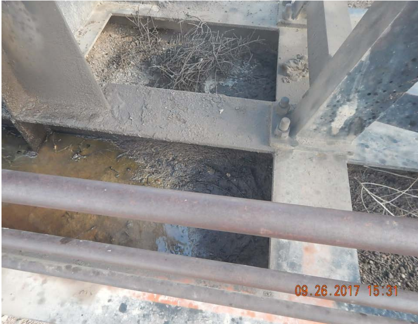
Photo 7: Stained soil, oily fluid at pump jack
