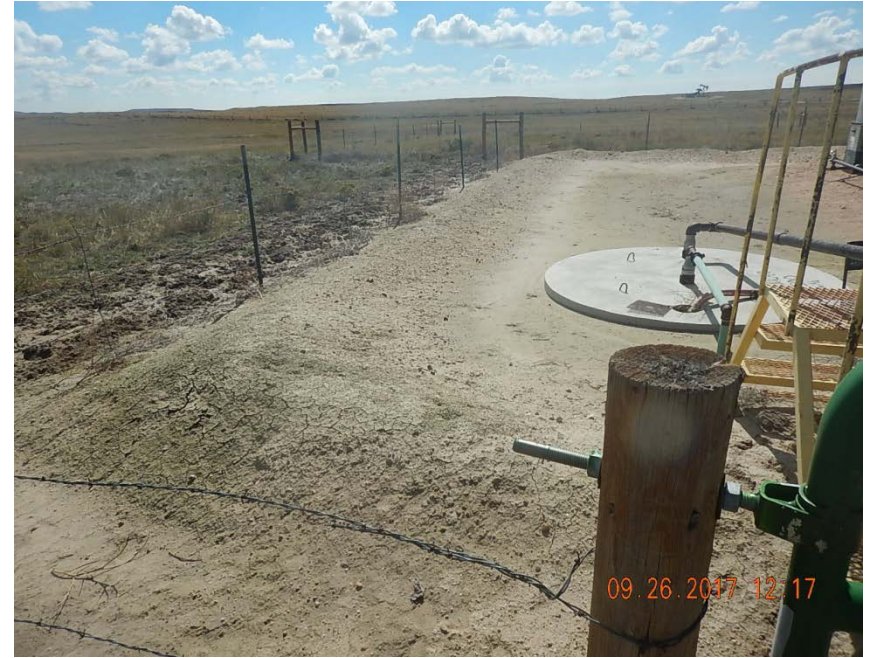
Photo 3: Low berms at tank battery
