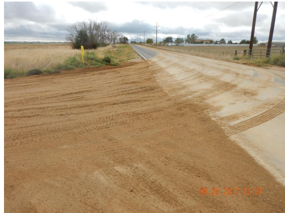
Photo 2: Photo taken from the access road and country road intersection to the southwest of the location, facing south. Photo shows vehicle tracking BMPs are no longer in proper function condition and need maintenance.
