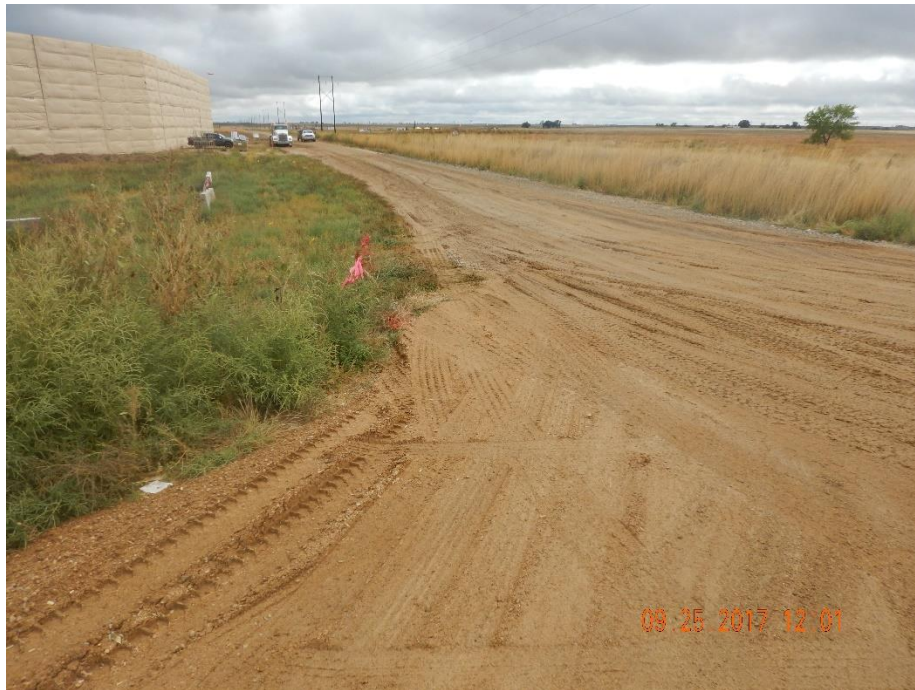
Photo 1: Photo taken from the access road and country road intersection to the southwest of the location, facing southeast. Photo shows vehicle tracking BMPs are no longer in proper function condition and need maintenance.
