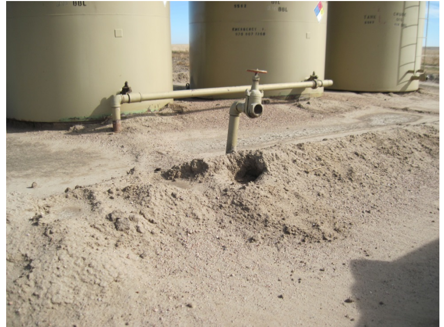
NEED CAP ON LOAD LINE AND HOLES IN BERMS
