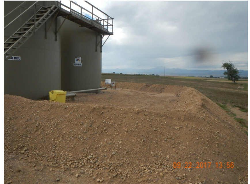
Crude oil tank berm on 9/22/17
