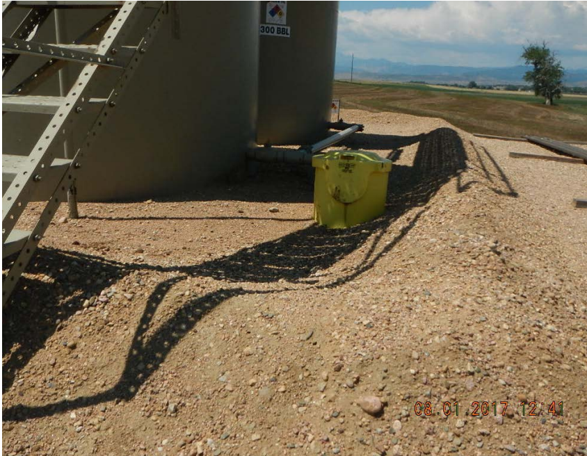
Crude oil tank berm on 8/1/17
