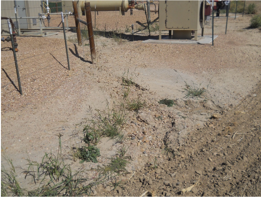
Discharge point from location washing out on southeast edge of location
