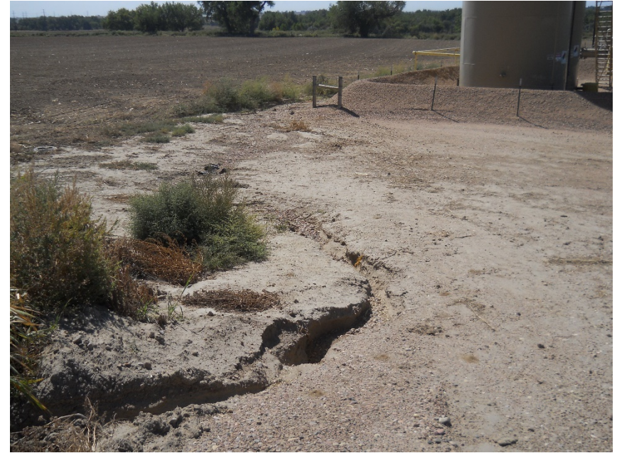
Location washing out from northeast edge of location entrance and running through east edge of location. Actively growing weeds on east edge of location need to be controlled
