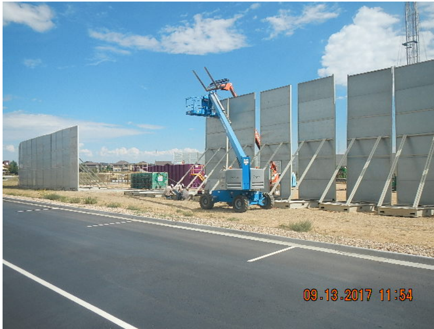
Phot of temporary sound walls being installed on west end of location photo taken from the west near playground at Aspen Ridge School
