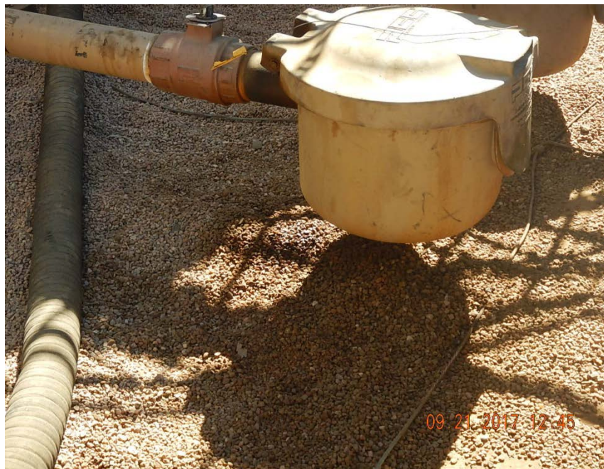
Photo 5: Stained soil at crude oil loadout.
