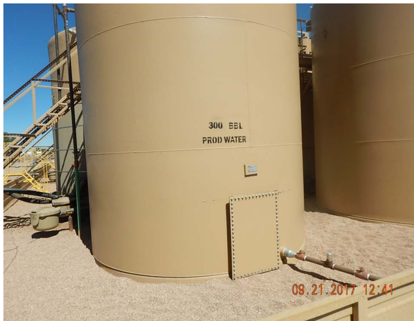
Photo 3: 300 bbl tank lacking safety placarding
