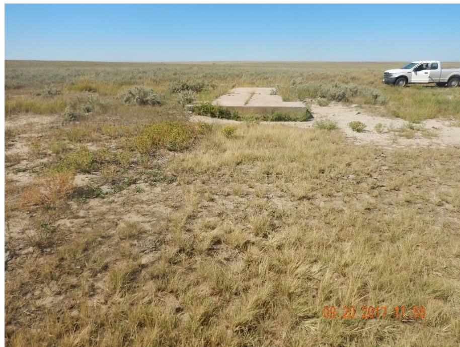
Photo 2: Photo taken from the east end of the location, facing west. Photo shows location does not meet reclamation requirements. Concrete pumping unit remains on location. Location has not achieved vegetative requirements.
