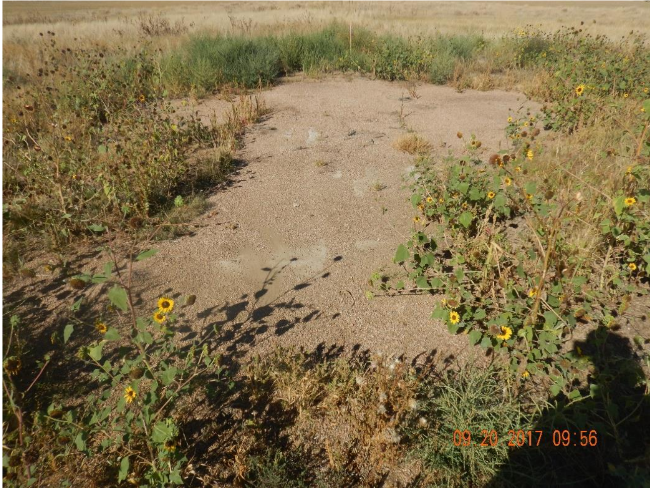
Photo 3: Photo taken north of the well location. Photo shows gravel had concealed the concrete pump unit base. This should also have been removed per reclamation requirements.
