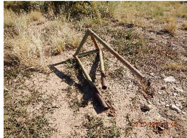
Photo 2: Damaged steel post and pole barrier.
