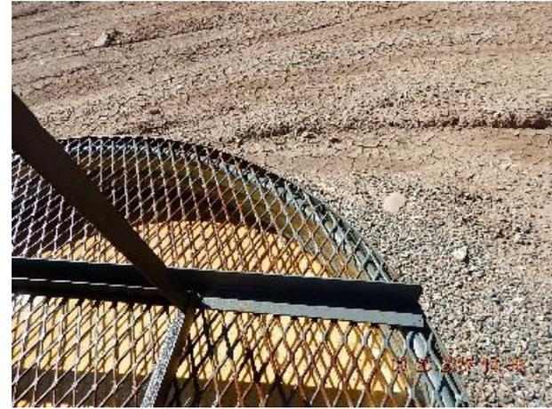
**Photo 6: Lube oil tank containment within 6" – 8" from top of containment.**
