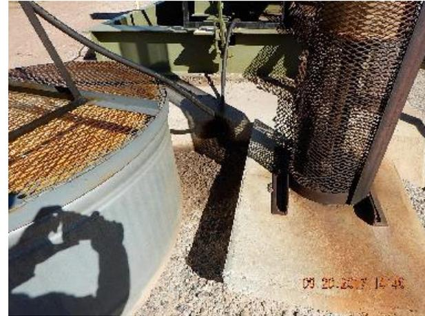
**Photo 4: Impacted soil and gravel at base of pump jack and containment.**
