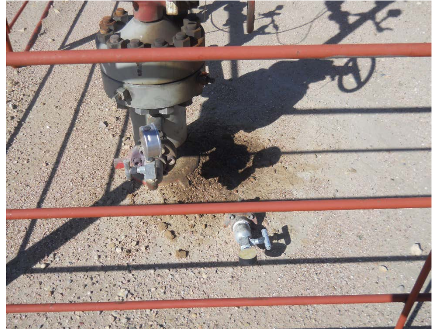
NC Farms 16-32...stained soil under master valve
