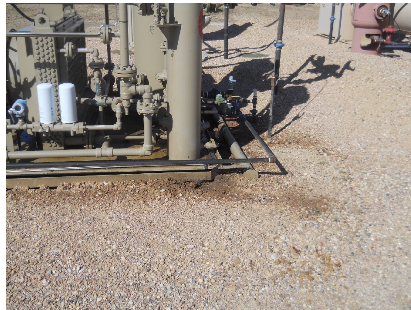
Stained soil around compressor skid
