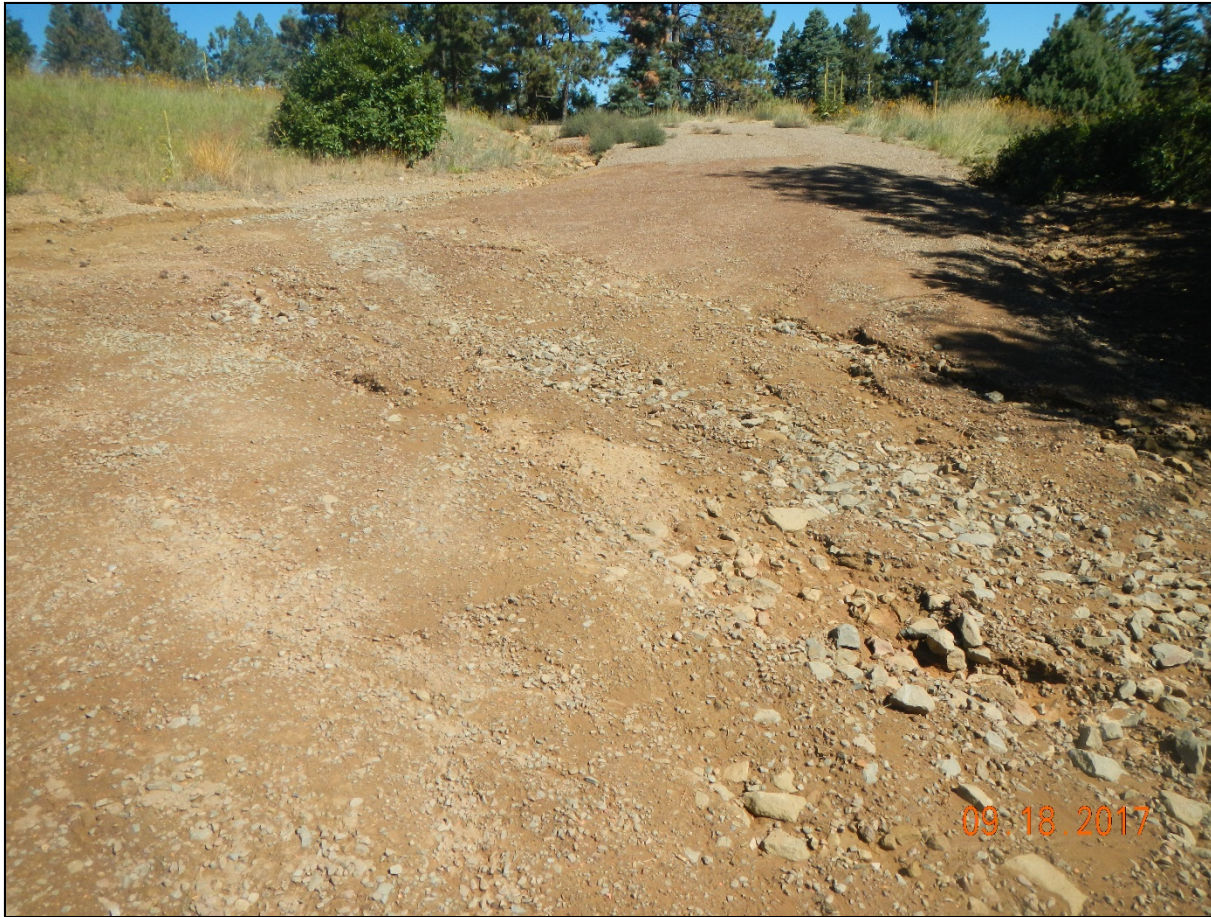
Photo 2. Facing northwest at the access road. There are signs of erosion occurring from recent storm events. This area was recently repaired and issues have already developed. A culvert may need to be installed to prevent erosion across the road.
