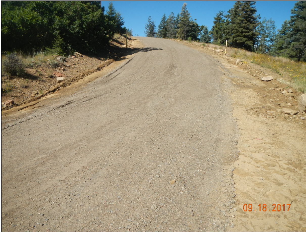
Photo 2. Facing west along the access road. Gravel was applied to the access road.
