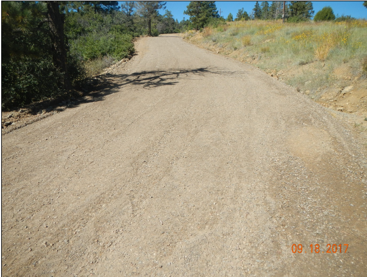
Photo 1. Facing west along the access road. Stormwater issues have been repaired.
