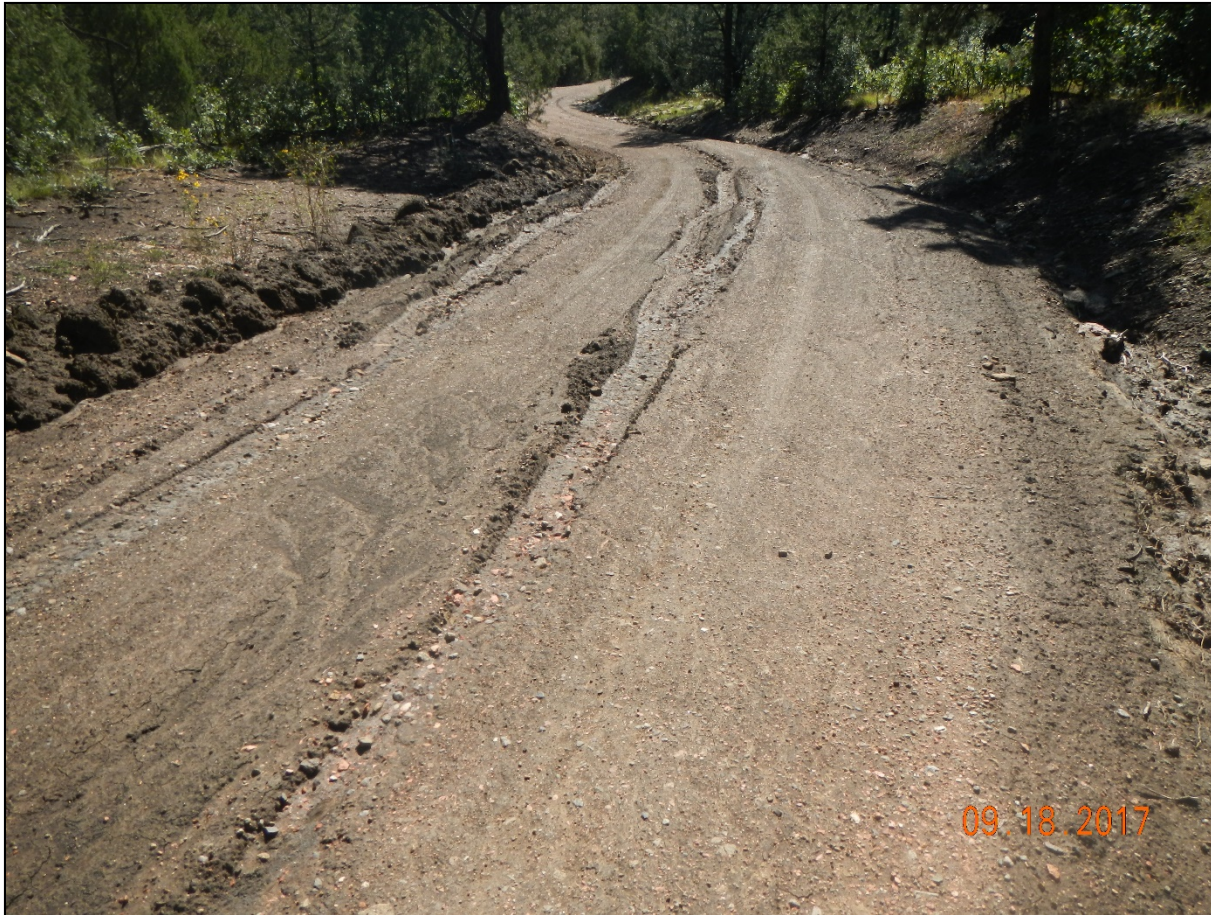
Photo 2. Facing southeast along the access road. This area was graded but does not appear to have much gravel. Stormwater issues may be more susceptible in this area.
