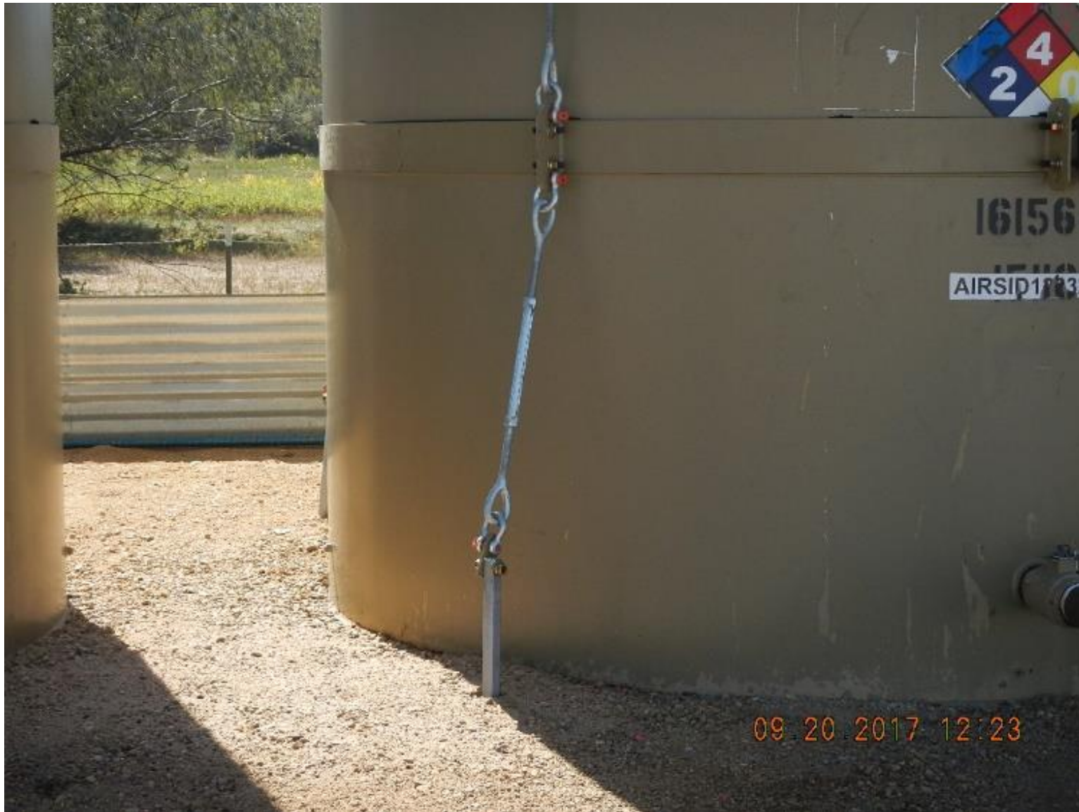
Crude Tank Flood Anchoring Location Number: 336259
