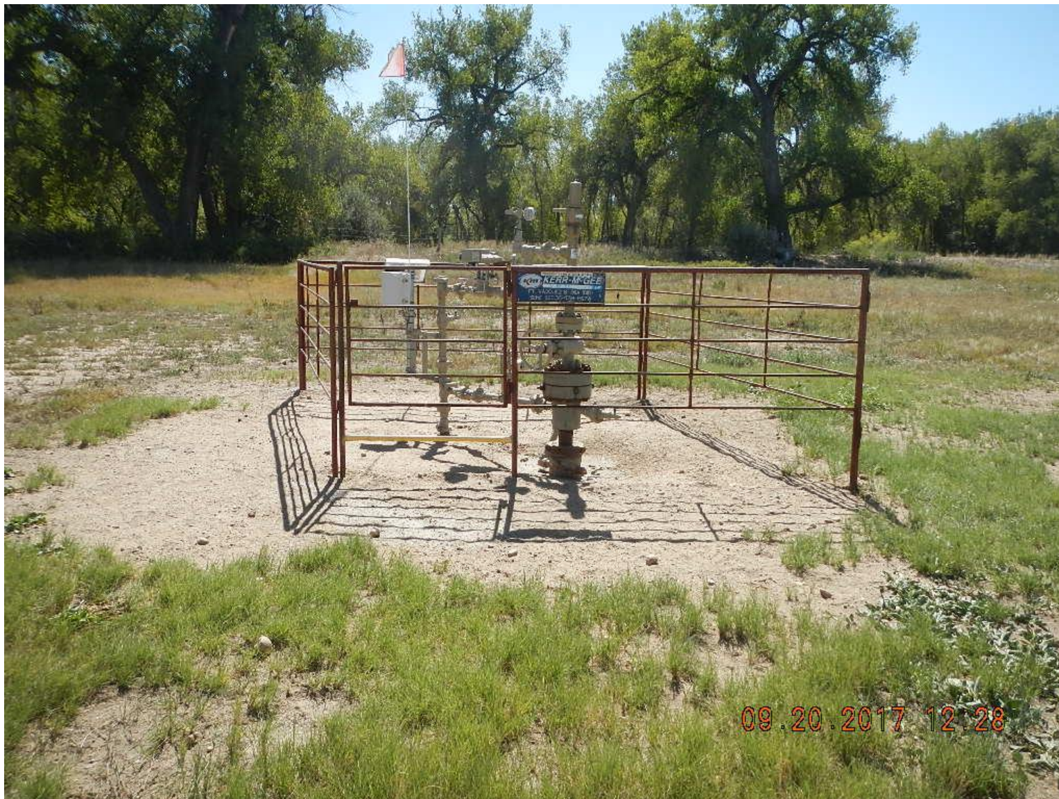
Wellhead HSR-FT Vasquez 8-36A Location Number: 336259
