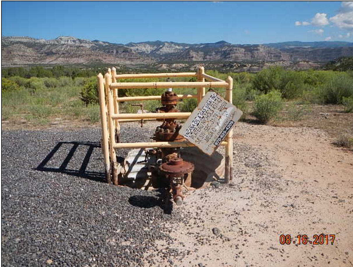
Photo 1. Well has been disconnected. Last MIT was on 10/6/2012
