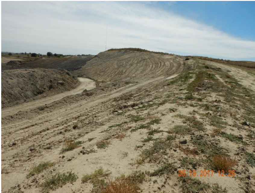
Photo 13. Photo taken from the western location, facing South. Cut slopes appear to be temporarily stabilized but will require additional long-term stabilization BMPs.
