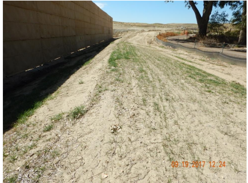
Photo 12. Photo taken from the northern location, facing Southwest. Areas constructed to be a berm have been seeded and mulched. Areas do not have uniform germination and may require additional stabilization.
