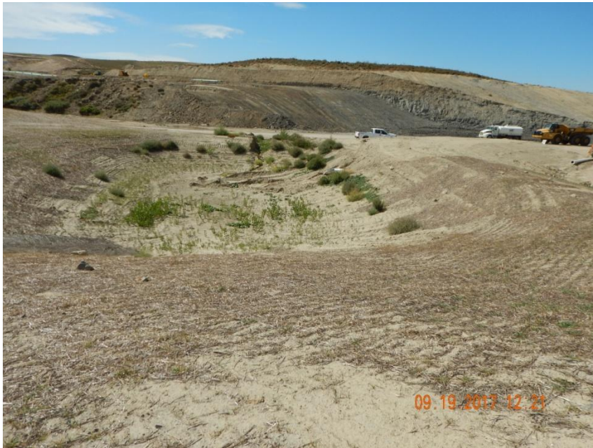
Photo 9. Photo taken from the southeast drilling pad location, facing South. Sediment basin has been installed with a stabilized outlet in conjunction with other stormwater BMPs.
