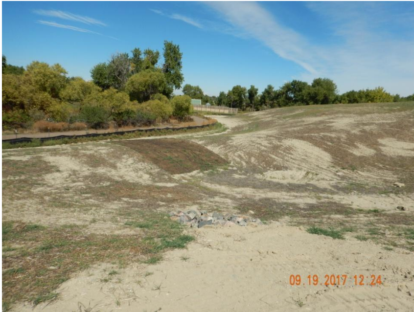
Photo 11. Photo taken from the northern location, facing North. Sediment basin has been installed with a stabilized outlet in conjunction with other stormwater BMPs. Areas do not have uniform germination and may require additional stabilization. May need additional reclamation activities for long-term self-sustaining stabilization.
