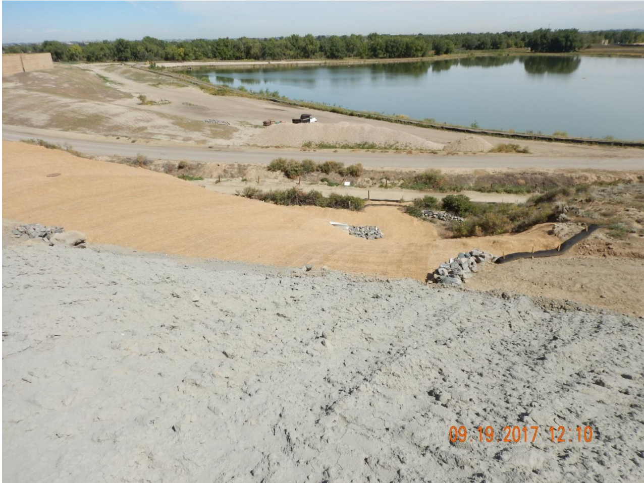
Photo 2. Photo taken from the eastern pipeline R-O-W, facing East. Erosion blanket, check dams and filtrex wattles have been installed along a portion of the eastern pipeline R-O-W.
