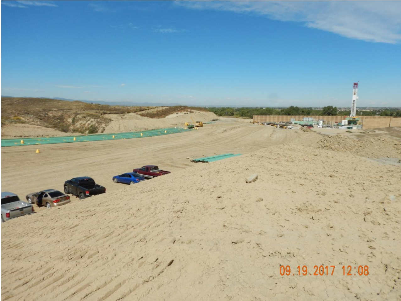
Photo 6. Photo taken from the eastern pipeline R-O-W, facing Northwest. Photo illustrates the flowline installation from the tank battery to the well location.
