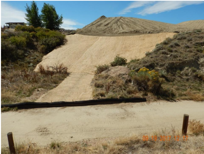
Photo 7. Photo taken from the downgradient slope of Photo 2, facing West. Erosion blanket installed along a portion of the eastern pipeline R-O-W.
