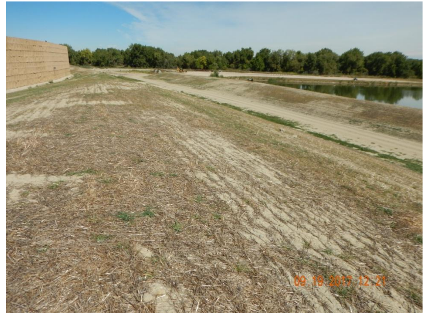
Photo 10. Photo taken from the southeast drilling pad location, facing North. Both the topsoil stockpile and other areas constructed to be a berm have been seeded and mulched. Operator indicated that a “TOPSOIL” sign would be placed to indicate the location of the topsoil. Areas do not have uniform germination but appear to be temporarily stabilized with mulch. May need additional reclamation activities for long-term self-sustaining stabilization.
