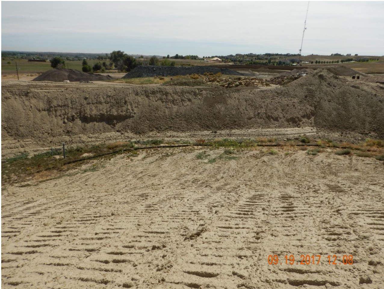
Photo 3. Photo taken from the eastern pipeline R-O-W, facing Southeast. It is unclear if some of the stockpiles are from oil and gas activities or from previous land use from the mining company. Silt fence has been installed at the toe of the slope.
