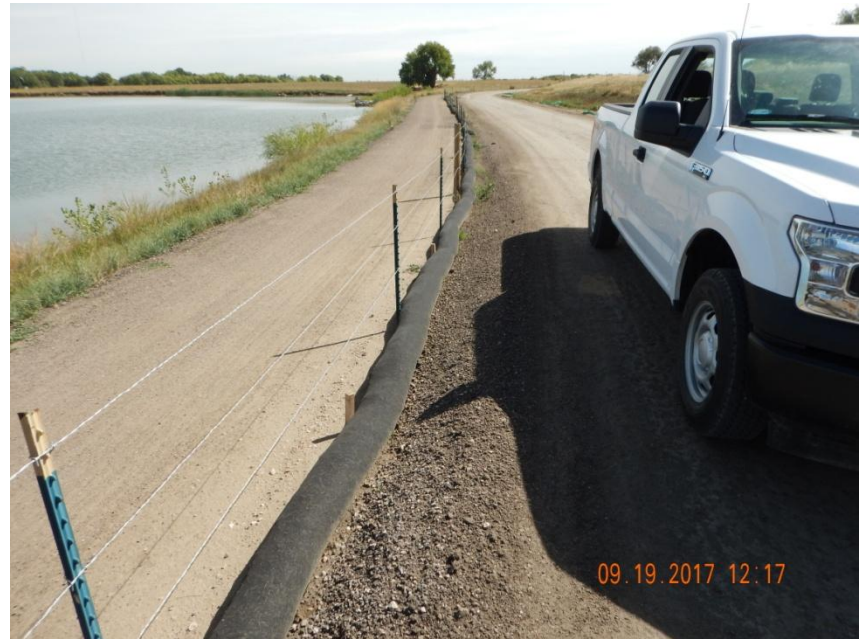
Photo 8. Photo taken from a portion of the access road, facing East. Filtrex wattles have been installed but do not appear to be properly staked. Silt fence was also installed along portions of the access road.
