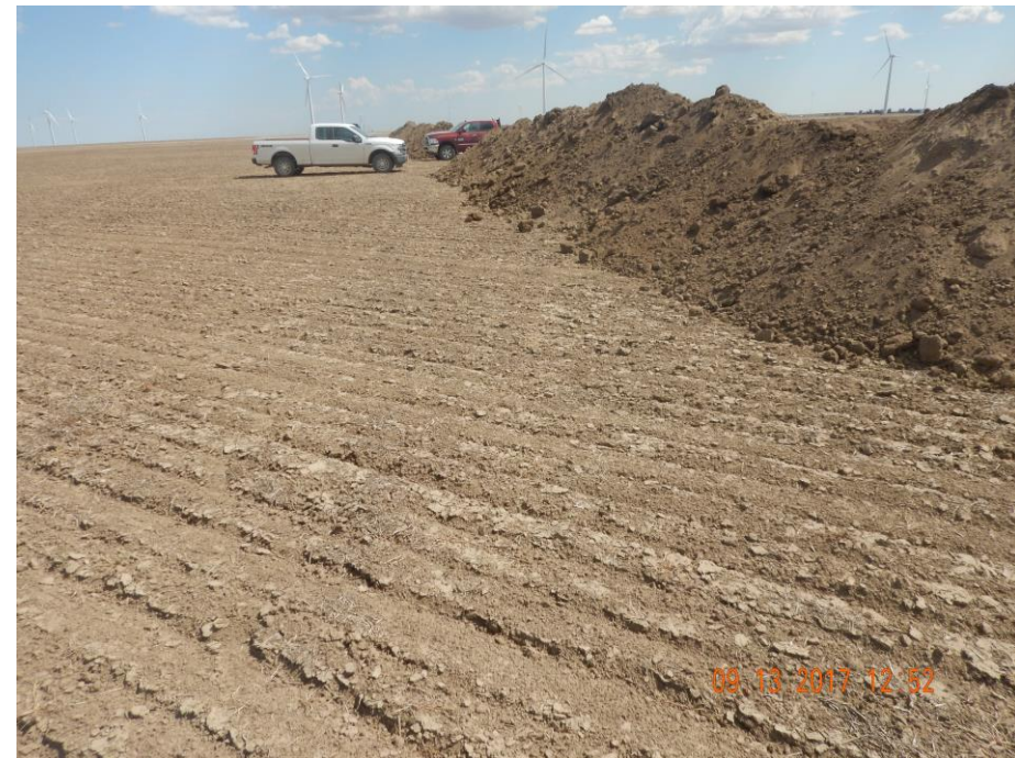
Photo 2: Photo taken from the northwest corner of the location, facing east. Photo shows stormwater and sediment control BMPs missing. Note: upon the arrival of inspector, the contractor constructing the location began to install surface roughening along the perimeter of the location. Stormwater and sediment control BMPs need to be installed prior to construction activities.
