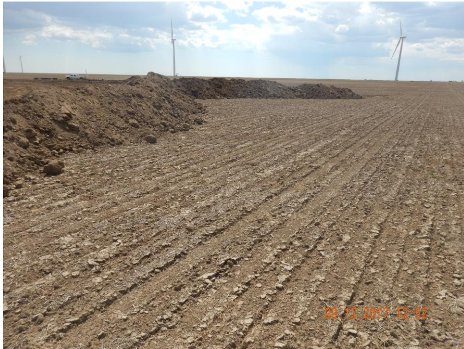
Photo 3: Photo taken from the northwest corner of the location, facing south. Photo shows stormwater and sediment control BMPs missing. Note: upon the arrival of inspector, the contractor constructing the location began to install surface roughening along the perimeter of the location. Stormwater and sediment control BMPs need to be installed prior to construction activities.
