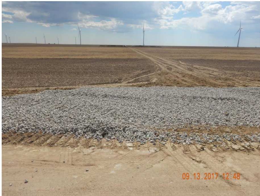
Photo 1: Photo taken from at the access road and country road. Photo shows rock had been placed as a vehicle tracking BMP.
