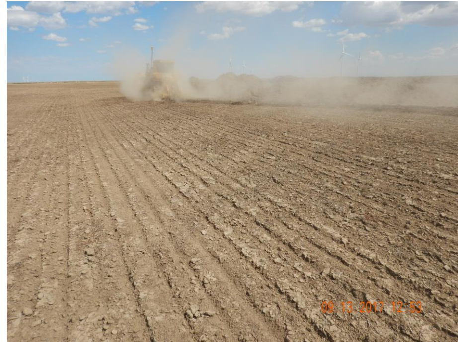
Photo 4: Photo taken from the west end of the location, facing west. Photo shows contractor constructing the location installing surface roughening along the perimeter of the location. Stormwater and sediment control BMPs need to be installed prior to construction activities.
