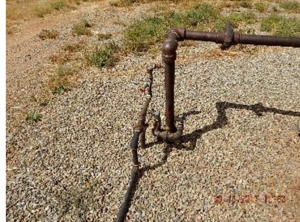
**Photo 4: Supply gas horseshoe at wellhead.**
