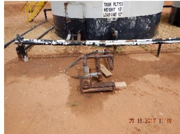
Photo 8: Recirculating line at oil tank battery.
