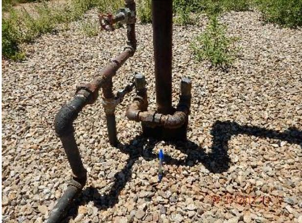
**Photo 3: Supply gas horseshoe at wellhead. Previous inspection.**
