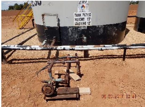
Photo 7: Recirculating line at oil tank battery. Previous inspection.
