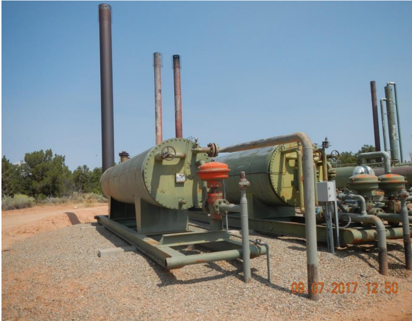
Facility separators and treaters.
