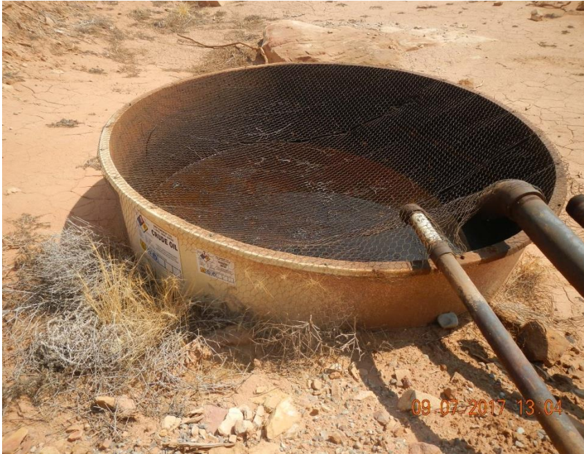
Wildlife netting on fiberglass tank.
