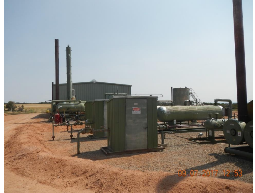
Meter runs, treaters, and separators
