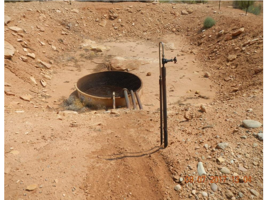
Open topped fiberglass tank inside pit.
