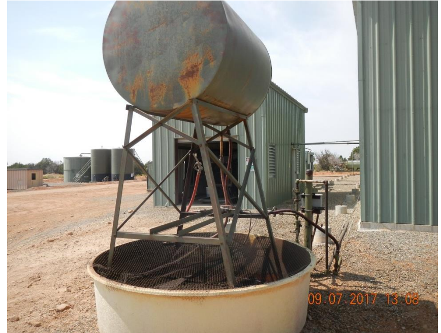
Secondary containment for fuel container.
