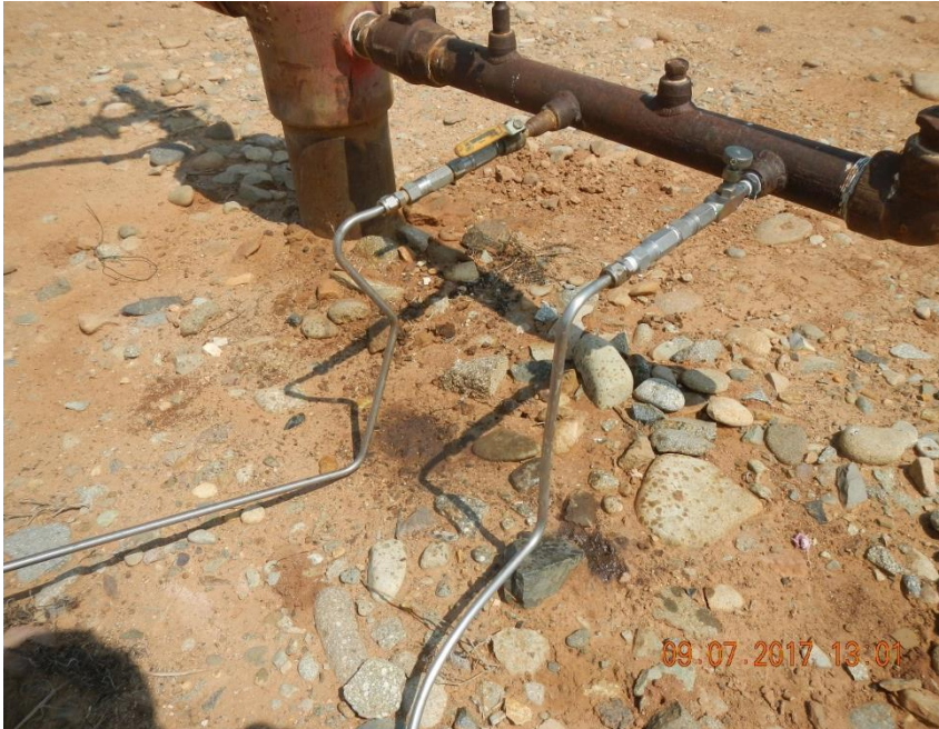
Leaking chemical injection fittings.
