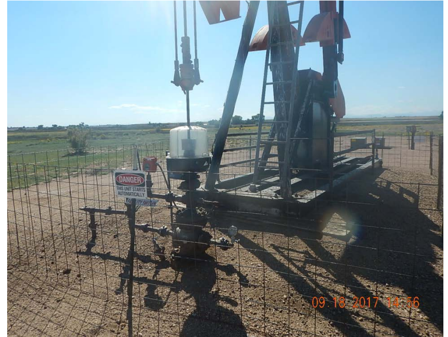
Photo 2: Wellhead looking SW
